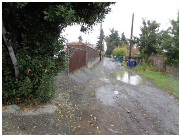
Trash, weeds and debris along an east alley edge below the church parking lot have been removed and replaced with a new gravel strip.
