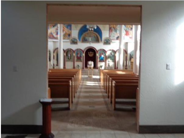
This photo shows an interior door opening that leads from the Narthex area to the Sanctuary. The existing door opening height was extended by over 1' to better accommodate processions out of the Sanctuary. The new doors will have stained glass and other accent features.
