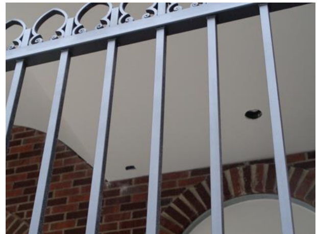
This is a close-up of an ornamental security bar panel that has been installed in smaller arched openings under the Narthex main entry overhang area.
