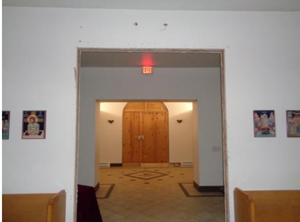
This photo is taken from the Sanctuary, and looks through the renovated Narthex area to the main entrance exterior door opening.
