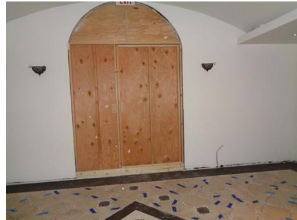
Above is the new exterior main entry door entrance opening that leads into the Narthex, with a temporary framed & sheathed cover over it. Since the time of this photo an interior lock has been added to supplement an exterior lock already in place at a temporary door that was constructed within that field framed opening cover. Batt insulation, covered with Visqueen is planned to be installed within the temporary cover to help maintain building heat as the outside temperatures drop. The temporary cover and door will be removed once the permanent exterior doors arrive.
