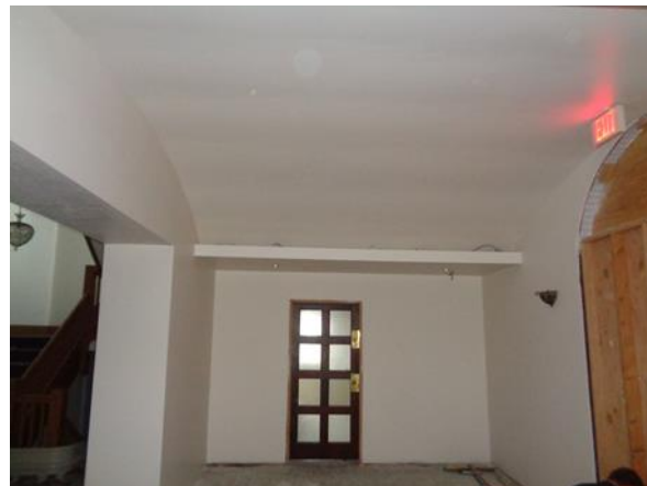
Above is a drywall ceiling in the south Upper Hall area recently patched and painted from a roof leak that occurred during the project. God willing, leaks over the Narthex will be a thing of the past.
