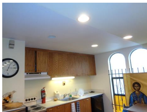
Above is a drywall ceiling in the south Upper Hall area recently patched and painted from a roof leak that occurred during the project. God willing, leaks over the Narthex will be a thing of the past.
