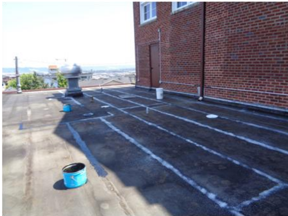
Above are some photos preventative roof repairs over the Dining Hall and Kitchen roof. Similar patches and repairs were done over the Upper Hall as well.
