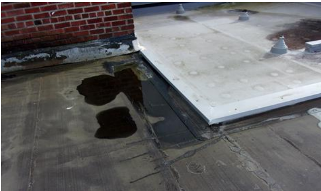
Above is the area of an Upper Hall roof leak that was discovered just beyond the new Narthex area roofing. Below is a close up of the patched area a few days later after some rainfall.
