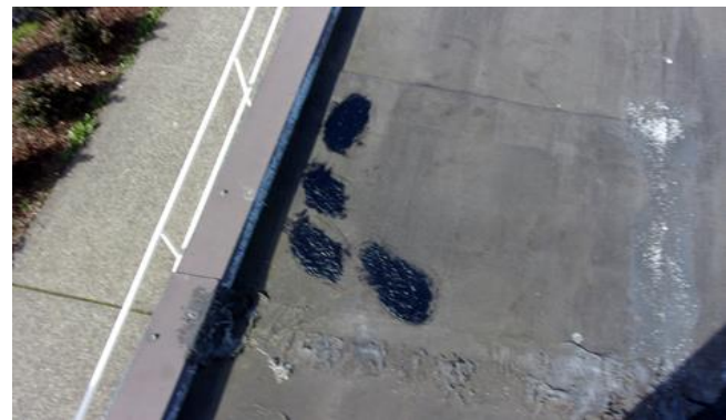
Above is where some staples were discovered at the Upper Hall roof edge facing Yakima Ave. The staples have since been pulled and their penetrations patched. Below is some standing water at the Dining Hall area roof.
