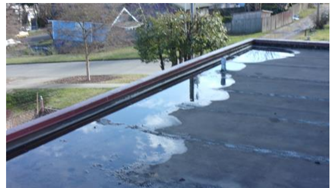
Above is where some staples were discovered at the Upper Hall roof edge facing Yakima Ave. The staples have since been pulled and their penetrations patched. Below is some standing water at the Dining Hall area roof.
