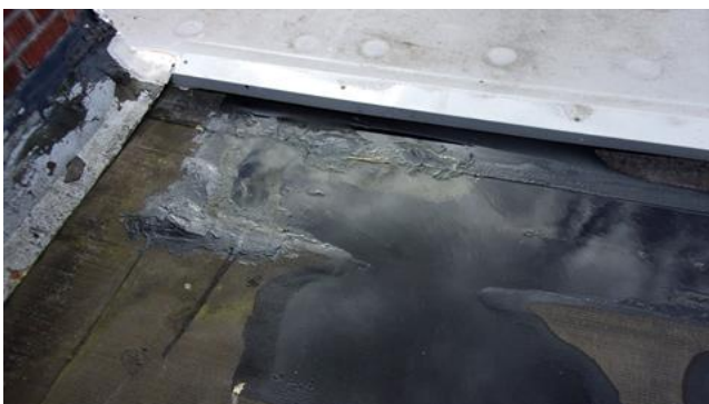
Above is the area of an Upper Hall roof leak that was discovered just beyond the new Narthex area roofing. Below is a close up of the patched area a few days later after some rainfall.
